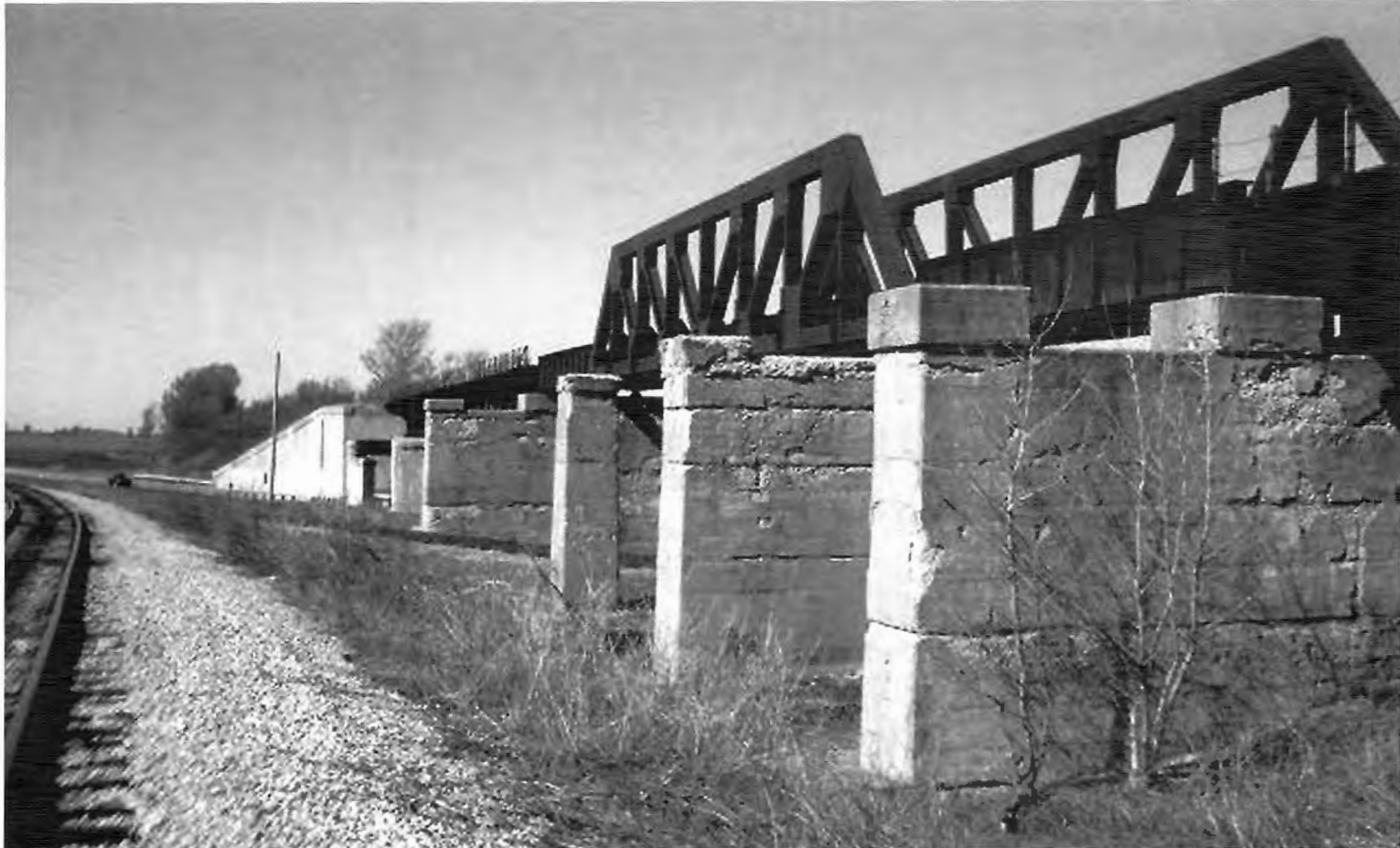
Although the embankment is only wide enough for a single track and that the wood-pile trestles are only one track wide, the concrete bridge supports are made wide enough for double track.
