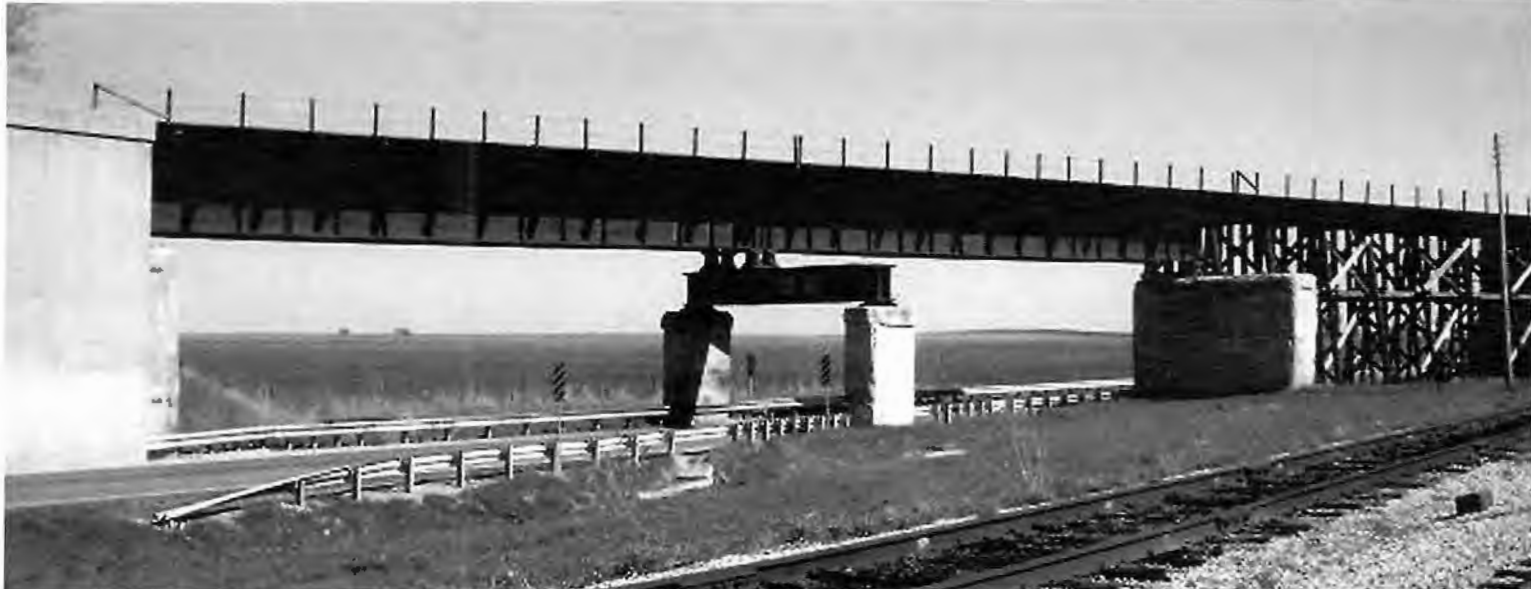
US Route 52 is a two-lane highway where it passes under the former Southeastern route. The highway passes between the piers of the center support of the deck truss section of the bridge.
