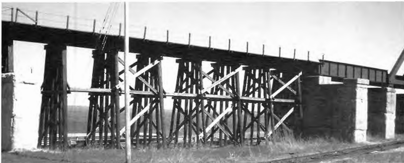
The steel girder sections of the bridge are connected by a short section of wood-pile trestle.
