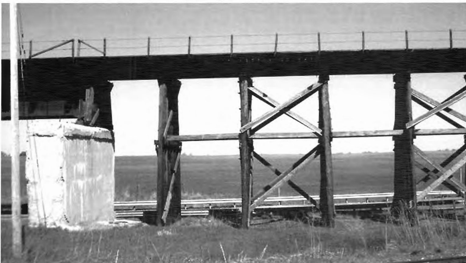
The wood-pile trestle sections are made with rather straight-forward construction. The bridge has a walkway with a wire guard fence.
