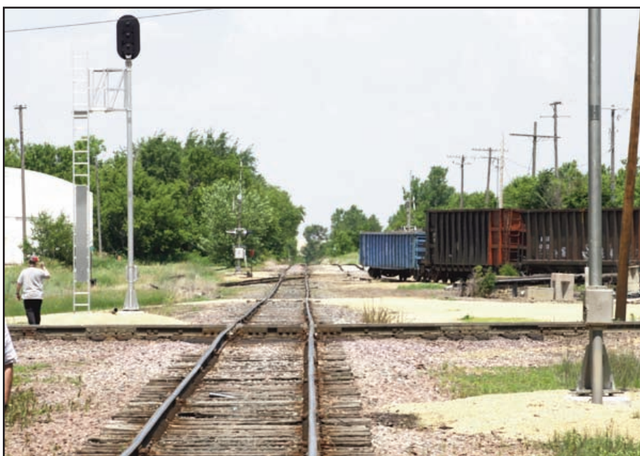
The crossing at Davis Junction, Illinois. Note the roadbed.
