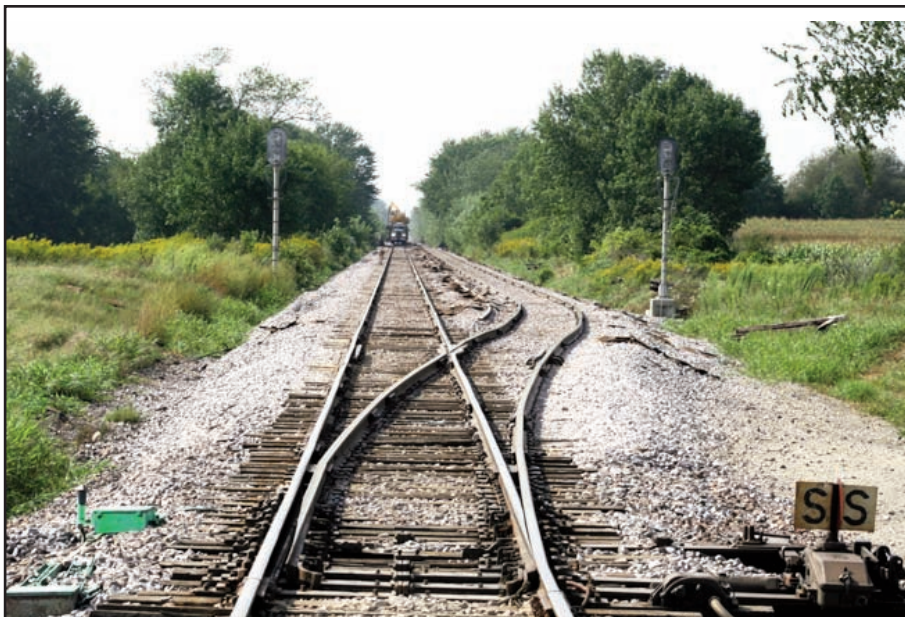
Below: A turnout on the UP/CNW mainline Adams Sub in Wisconsin. Note the shape of the roadbed.
