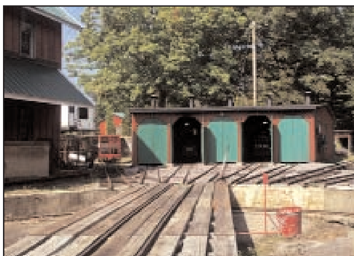
Looking back across the turntable at the roundhouse. The SLHTS was given a behind-the-scenes tour of the roundhouse, engine shop and car shops.
